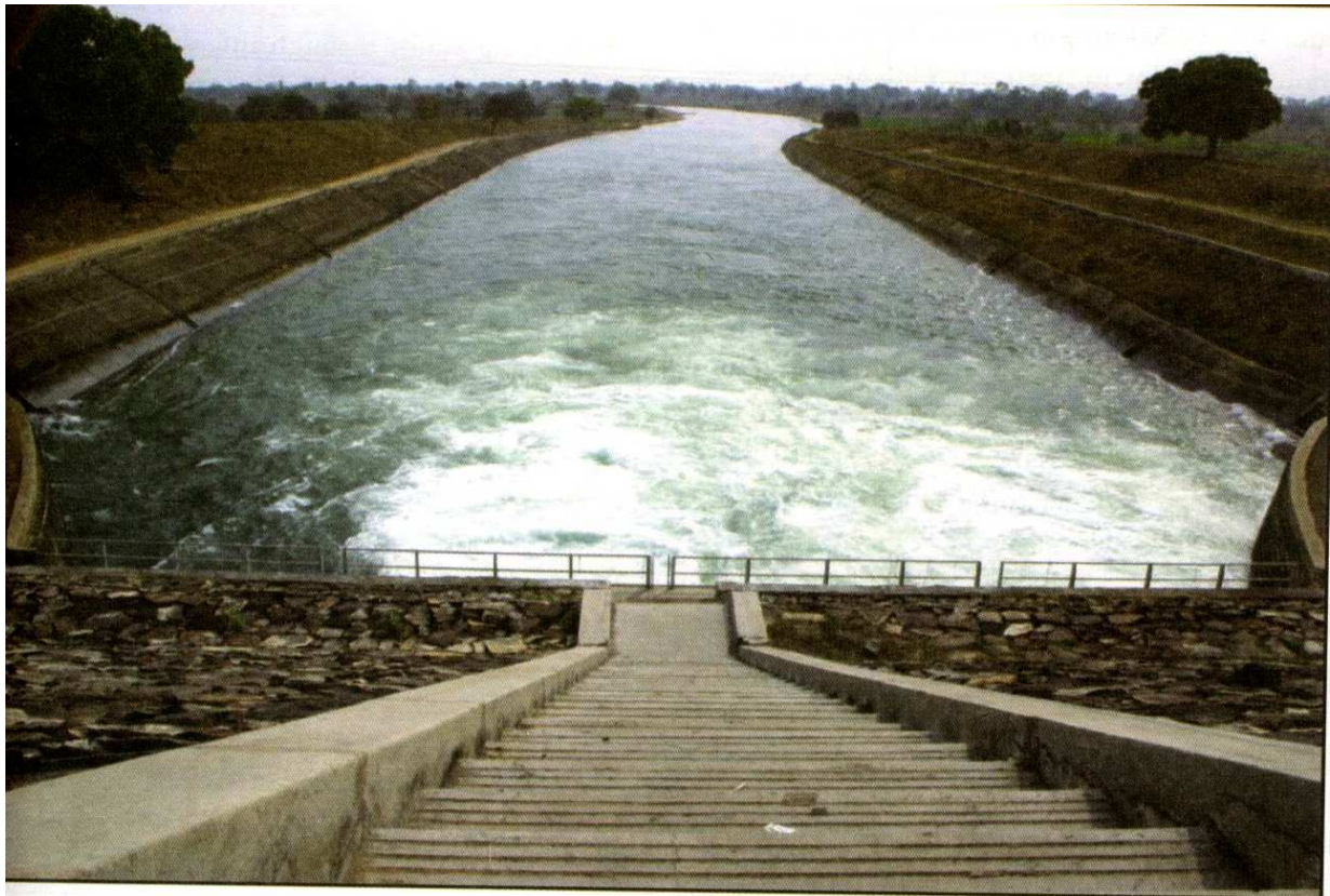
Aerial view of Baragada Main Canal (Hirakud Dam Project)
