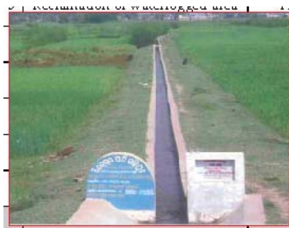
Field channel work at Balisahi of Kendrapara Canal System (Mahanadi-Delta Stage-I)
