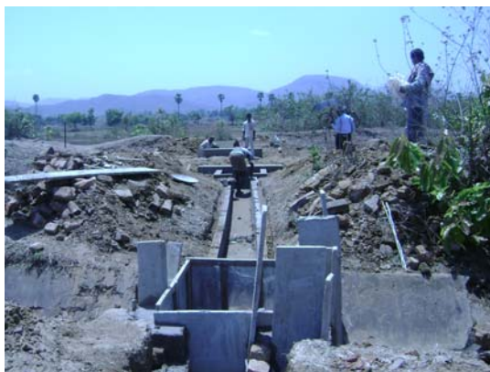
Field channel construction in progress in Madhyakhanda (Kuanria)
