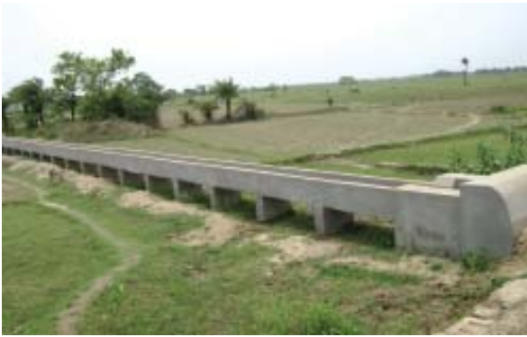
Field channelwork at village of Patamundai Canal System (Mahanadi-Delta Stage- I)
