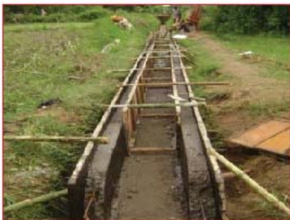
Field channel construction work under progress in Tikarapali (Budhabudhiani)
