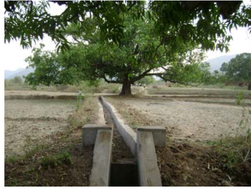
Field channel in Hatiguda (Daha)
