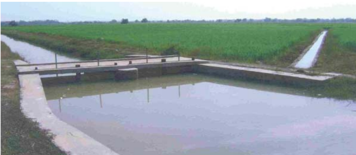
Field drain at Nilka to Bina Pinjara (Salandi Right Canal)
