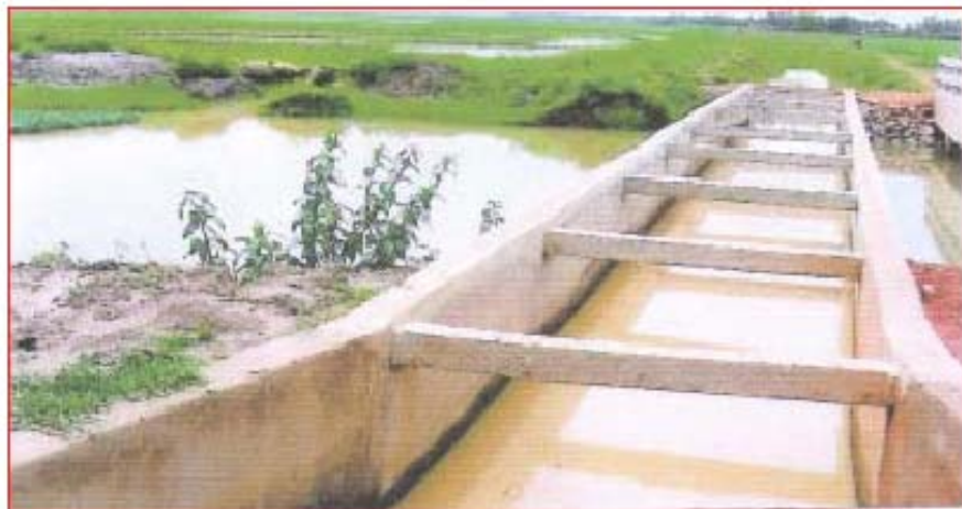
Canal aqueducts across Govari drainage system (completed RIDF-XII)
