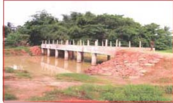
Pile Foot Bridge over Junei drainage channel (completed under RIDF)
