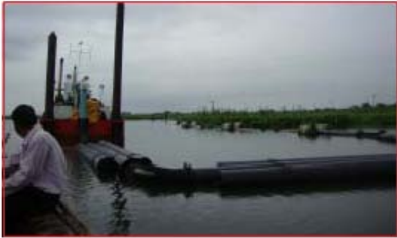
Improvement to Bahilpur drainage (dredging work in Progress under FMP)
