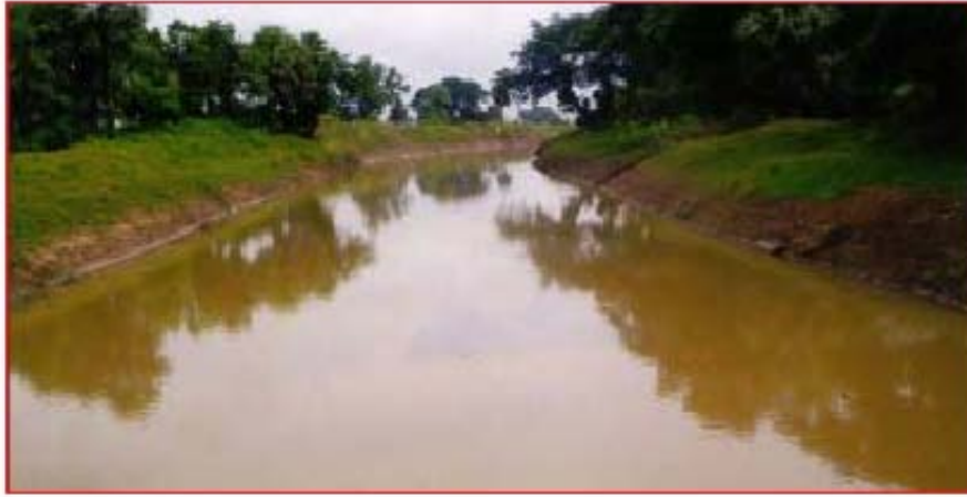
Chotagenguti drainage channel (work completed under FMP)
