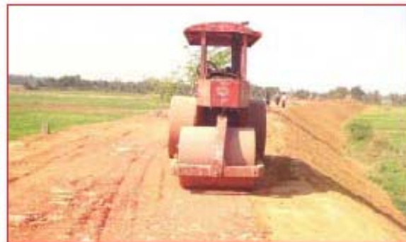
Bank protection at Sribantapur (work in under RIDF-X)
