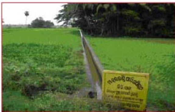
Field channel constructed by members of MAA Harachandi Pani Panchayat
