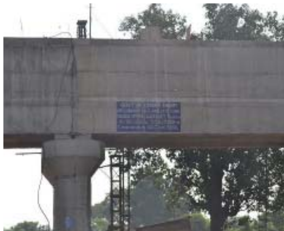
Upper Indravati Project (Sagada aqueduct)
