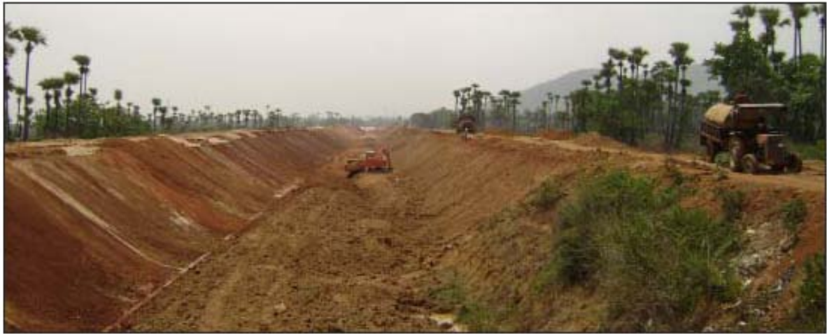
Subernarekha (Canal excavation in progress)
