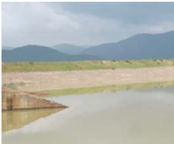
Lower Indra Project (Reservoir impounding view)
