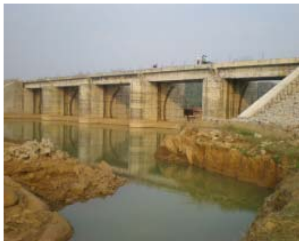
Titilagarh Irrigation Project Spillway
